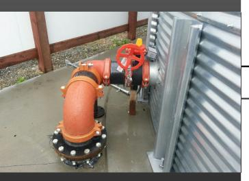
All required fitting sand appurtenances are available for SteelCore® Fire Tanks as per NFPA-22. Suction Nozzles, Anti Vortex Assemblies and more. You can rest assured that your tank meets NFPA-22 equivalent.
